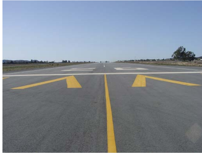
Relocated Threshold Markings
