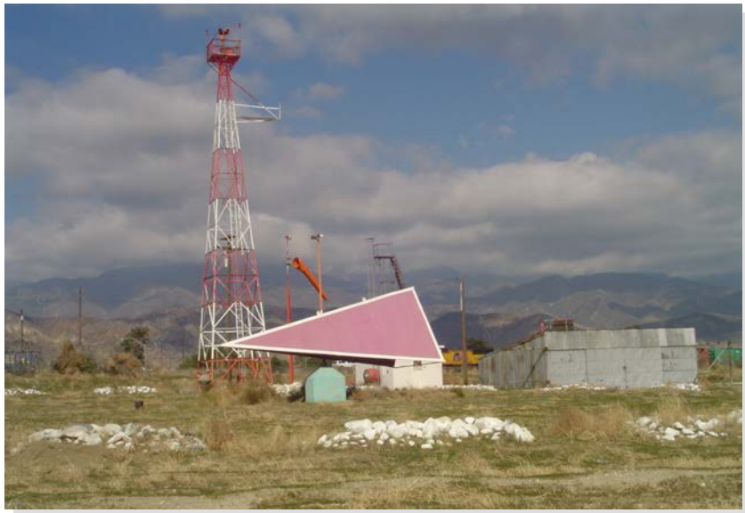
Beacon, Lighted Wind Cone, Tetrahedron & Segmented Circle
