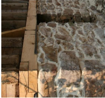
BARN BOARD AND BATTEN SIDING WITH FIELDSTONE FOUNDATION/BASE FOR TOWER
