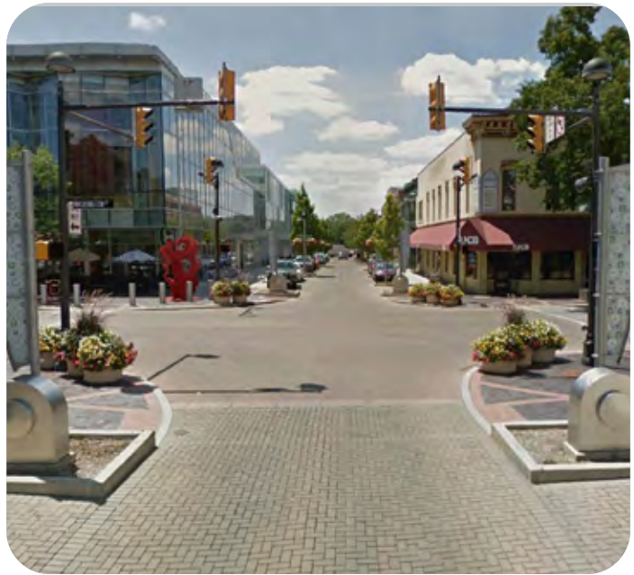
⑦ Raised Intersections- Changes environment from car to pedestrian orientation
