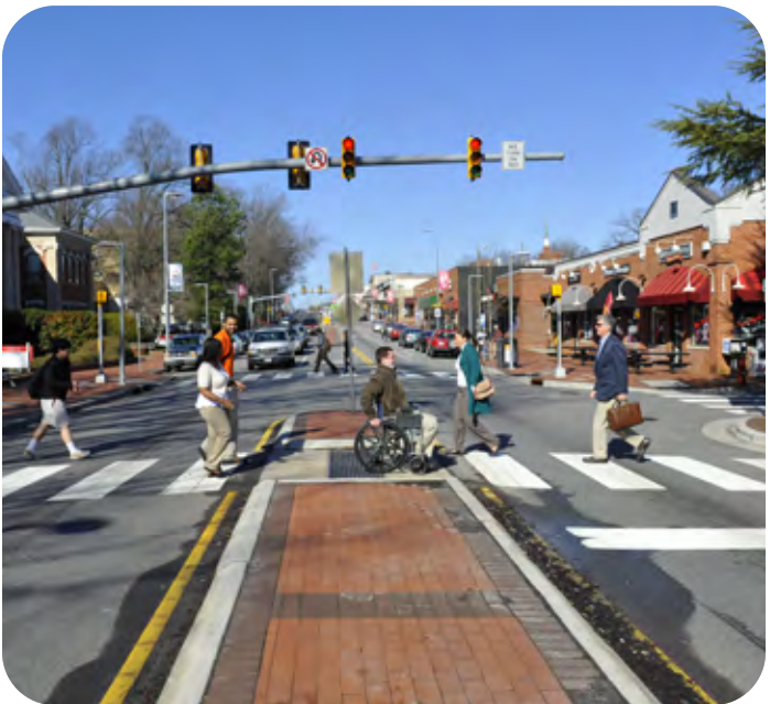
⑥ Midblock Median- Reduces exposed crossing distance and creates safe waiting space.
