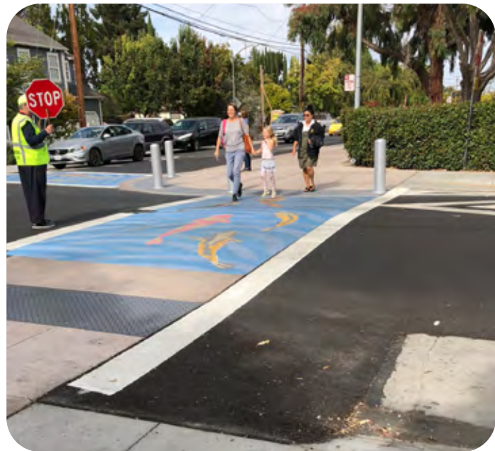
④ Raised Crosswalks- Connects pedestrians at sidewalk height while slowing vehicles
