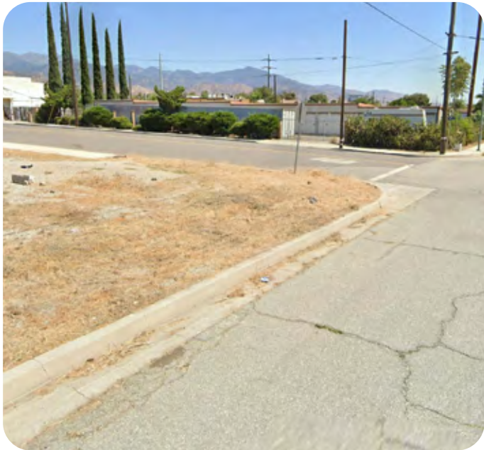
① Incomplete Sidewalk and Curb Ramps Not ADA Compliant
