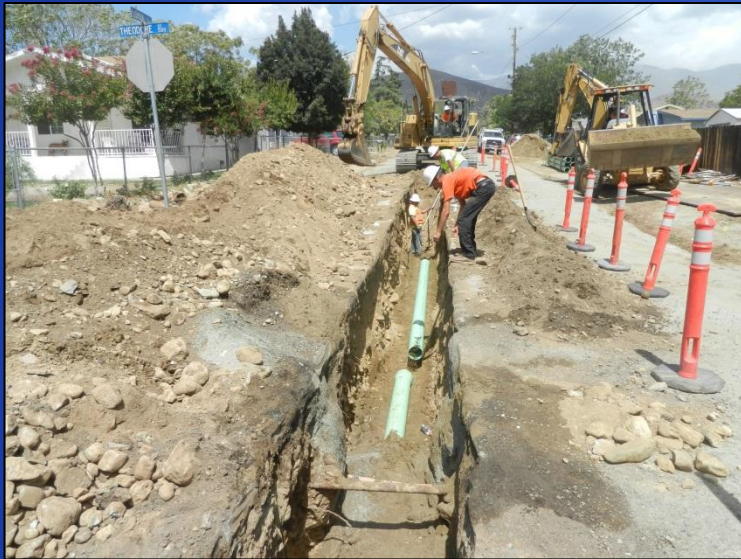
Before and After: Florida Street Sewer Main Replacement
